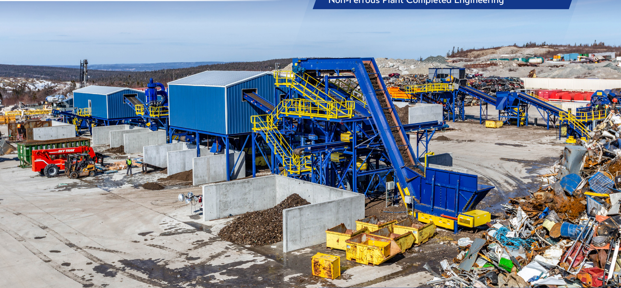
Non-Ferrous Plant Installed
