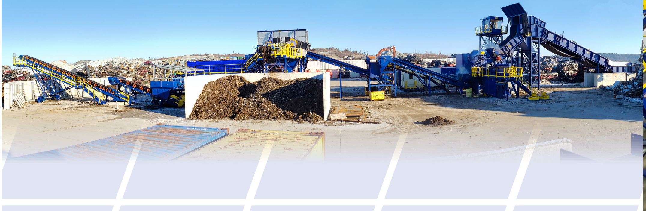
M6090 Modular Shredder Plant Installed
