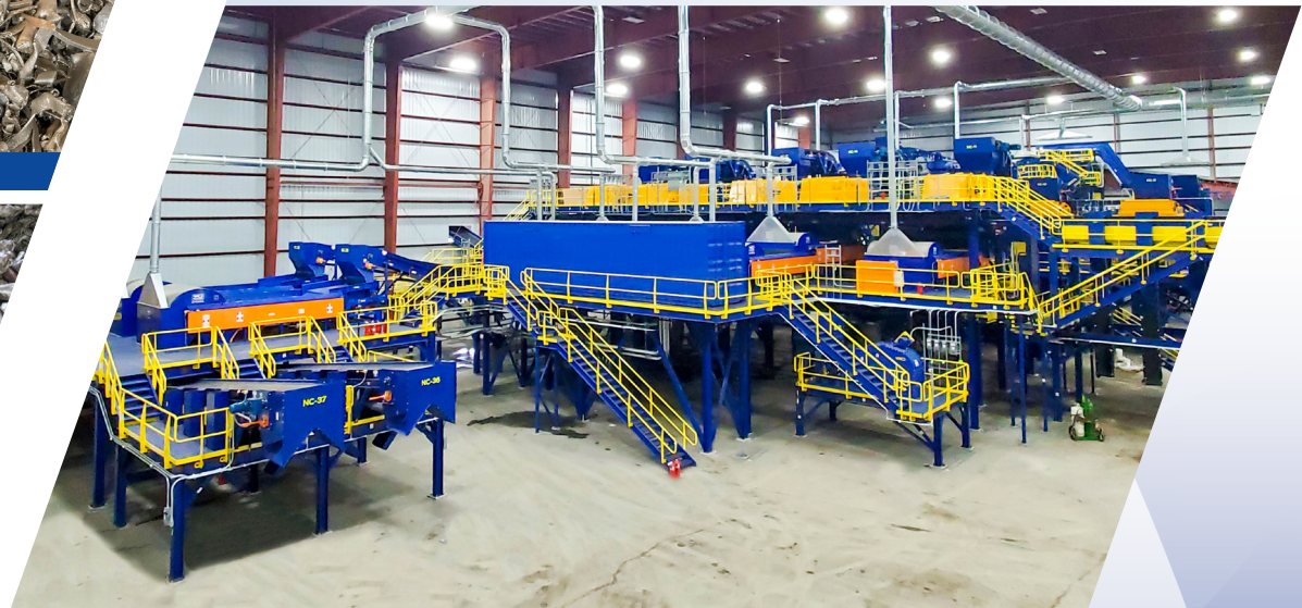
70 TPH Non-Ferrous Recovery Plant
