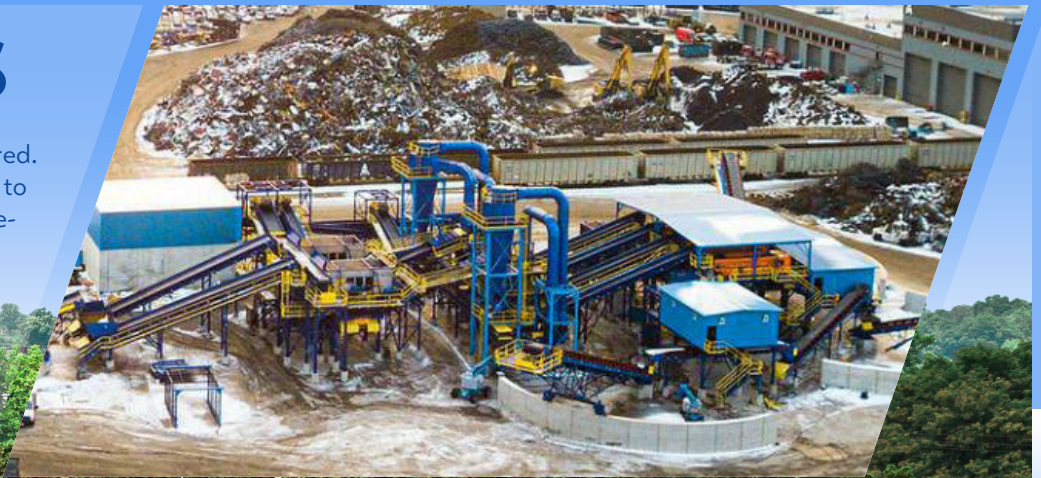
400+ TPH Ferrous Cleaning System (Low Copper)
